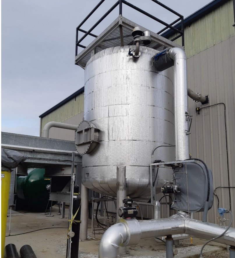
Hydrogen sulfide removal vessel at the Kelowna Biogas Plant (2021)
