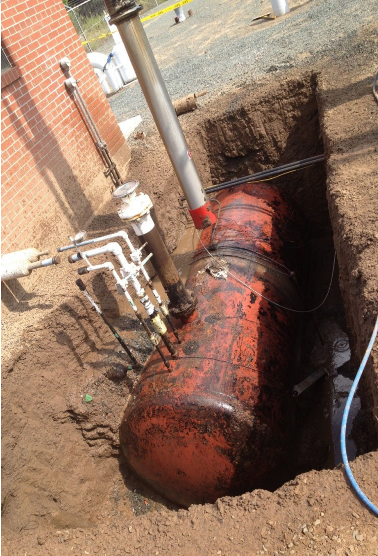
Draining odorant from the tank
