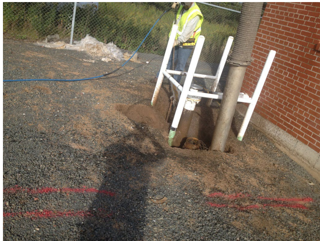
Hydrovac excavation
