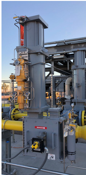
Ball Valve Regulator with Spring Return Actuator and PID Pilot Controls
