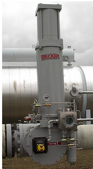
Ball Valve Regulator with Spring Return Actuator and Electro-Pneumatic Positioner
