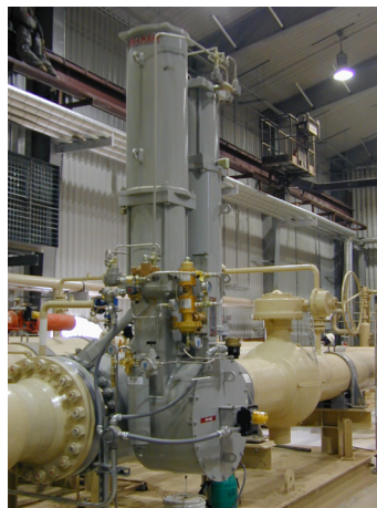
Compressor Surge Control Ball Valve Regulator with Spring Return Actuator and Pneumatic Positioner
